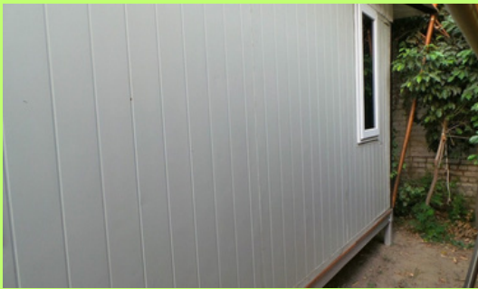
Tent side Walls in 50mm insulated Panels
